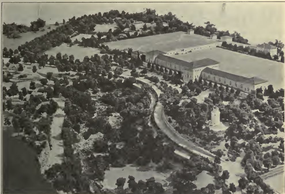
MODEL OF GROUNDS OF BALDWIN FILTRATION PLANT AND RESERVOIR, PREPARED FROM LANDSCAPE ARCHITECTS' PLANS
